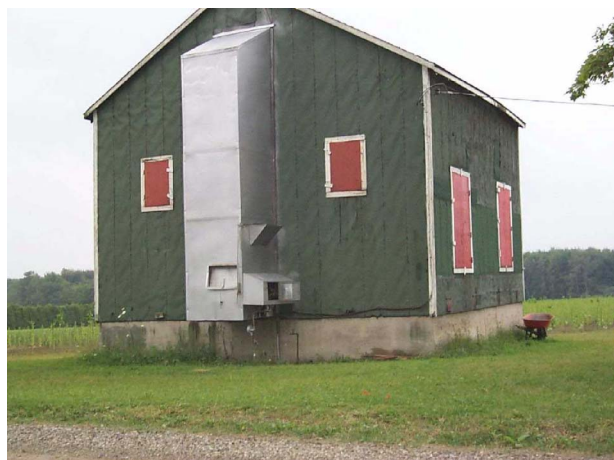
Figure 3 A downdraught kiln with an external natural gas burner.
