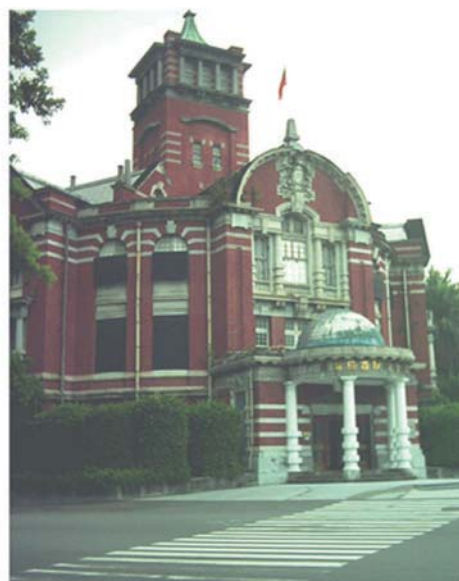
Historical landmark– The Monopoly Bureau building with more than a century of dominance (shown in cover picture)
